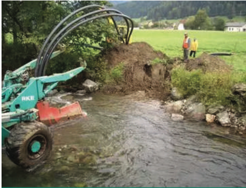
Laying pipes through watercourses
