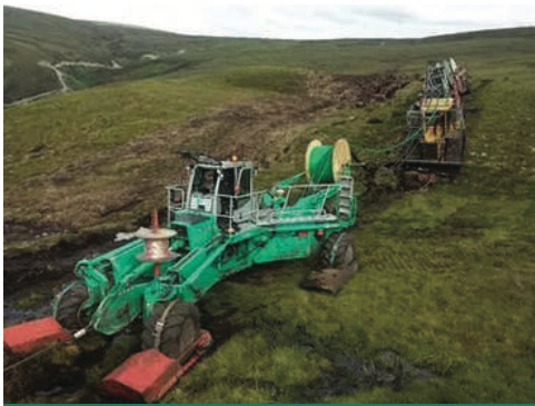
Laying system in mud and bog areas
