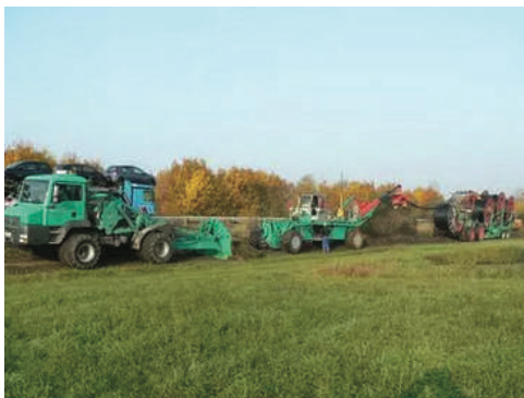
Laying of power cable
