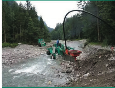
Laying system on rocky ground
