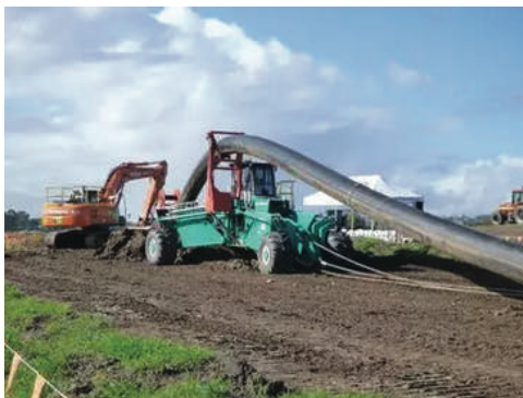
Laying of gas- and waterpipes
